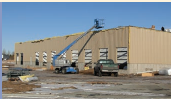
Frito Lay building under construction
